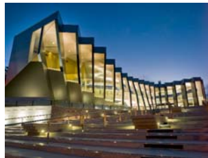
Page 38-39 STP254 Wall luminaires/recessed Medical Research Centre Canberra (AUS)
