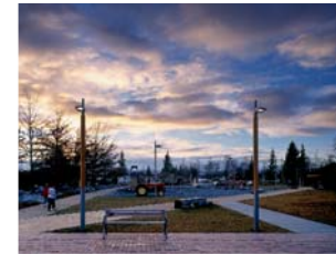
Page 88-89 PFL230 [S] Street and area lighting Twizel Town Centre Twizel (NZ)
