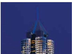
Page 140 FLC260 [EE] Projectors Highmark Office Building Pittsburgh (USA)
