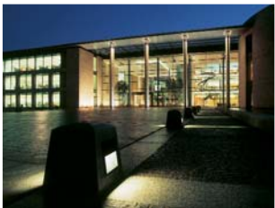
Page 34 QR1304 Wall luminaires/recessed Royal Bank of Scotland Edinburgh (UK)
