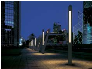
Page 60-61 LSP444 Light columns IFC Mall Hong Kong (PRC)
