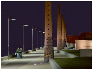
Page 74 PFL260 Street and area lighting Drift Park Rhyl, North Wales (UK)
