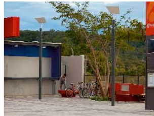
Page 64 LCI440 Light columns Varsity Lakes Queensland (AUS)
